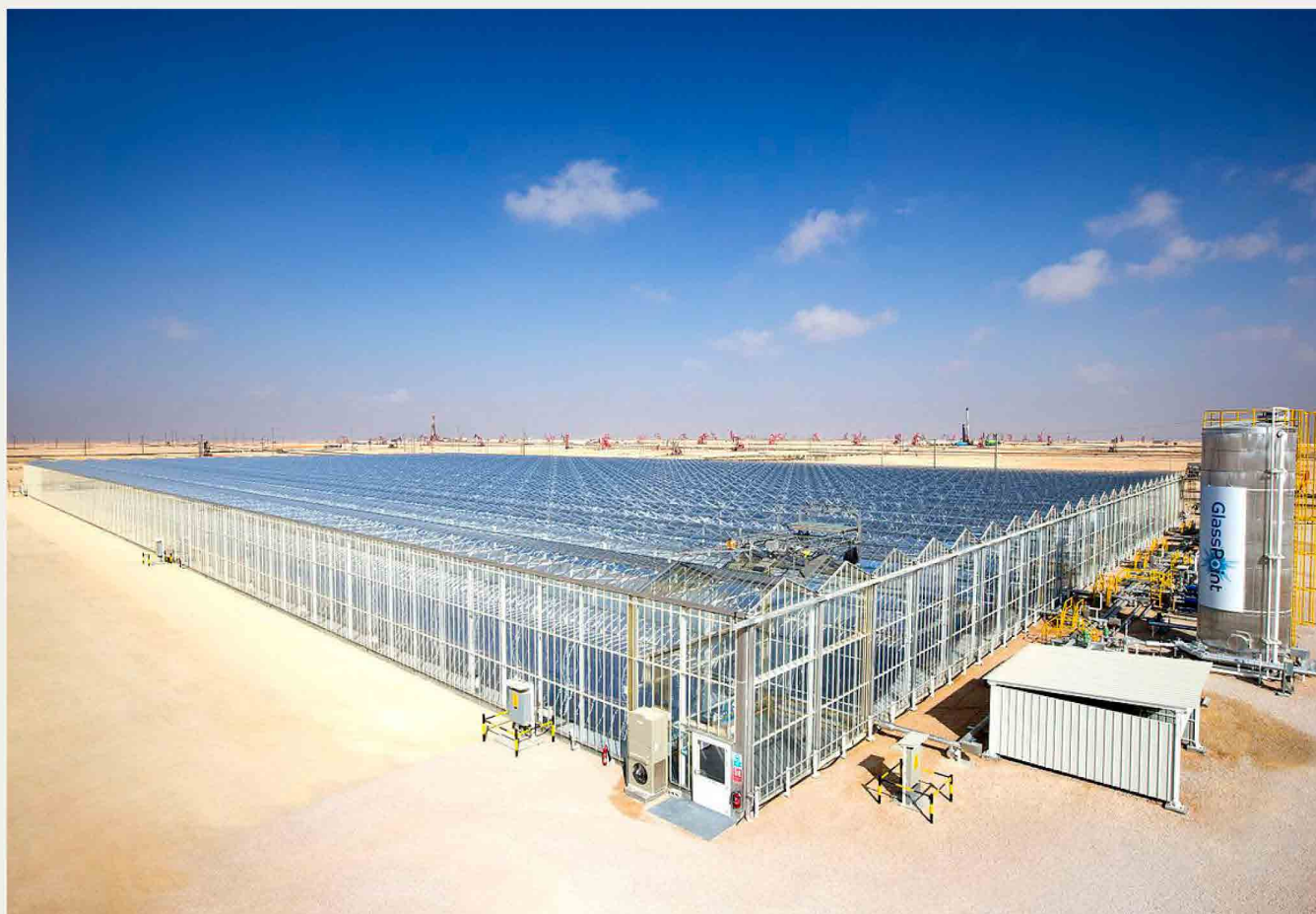
Oman's GlassPoint Amal EOR Project that utilises CSP to generate steam for EOR, Amal, Oman ( https://commons.wikimedia.org/wiki/File:GlassPoint_Amal_EOR_Project.jpg )
